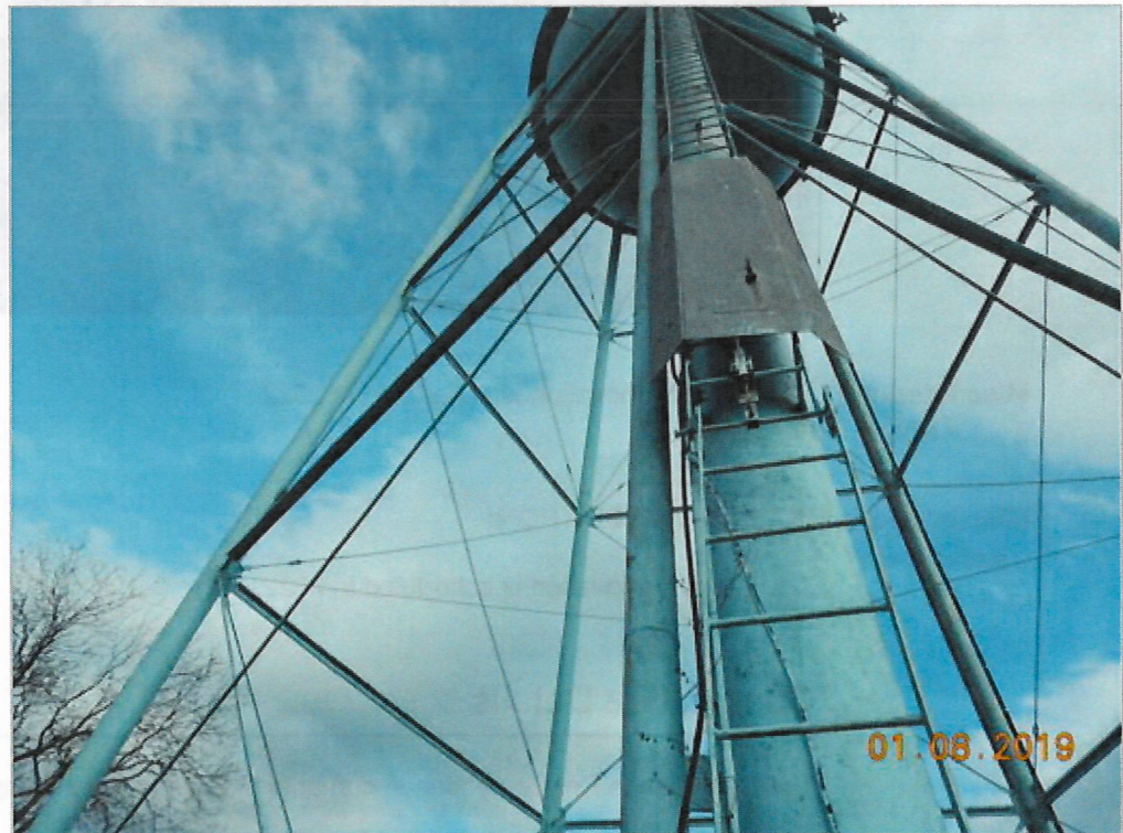
Trespass Protection Picture
