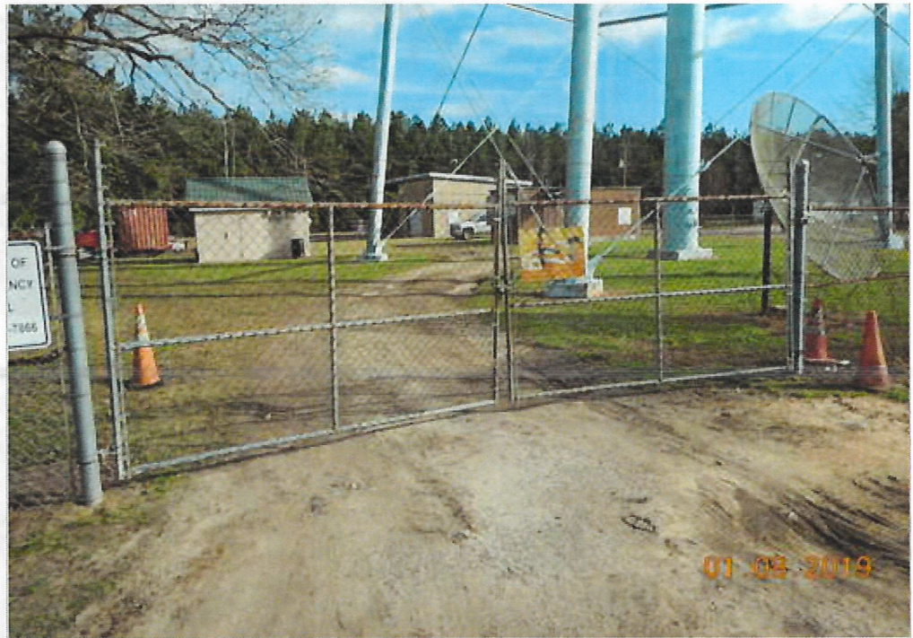
Site Access Picture
